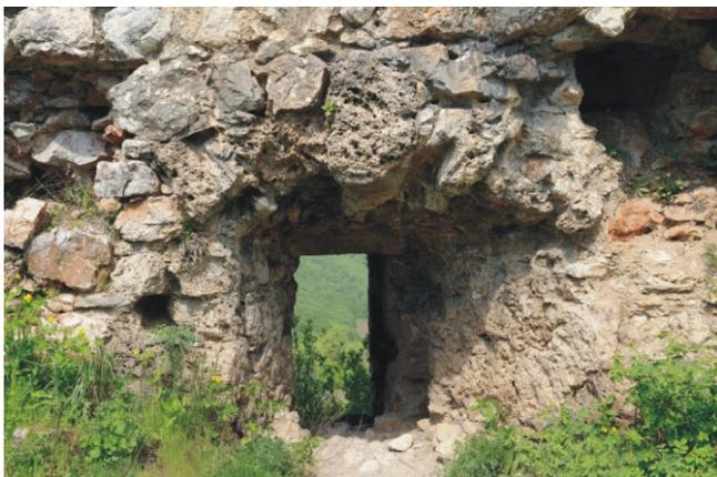
Fig. 1. Lintel constructed of resistant tufa facies in the medieval castle at Turňa nad Bodvou
