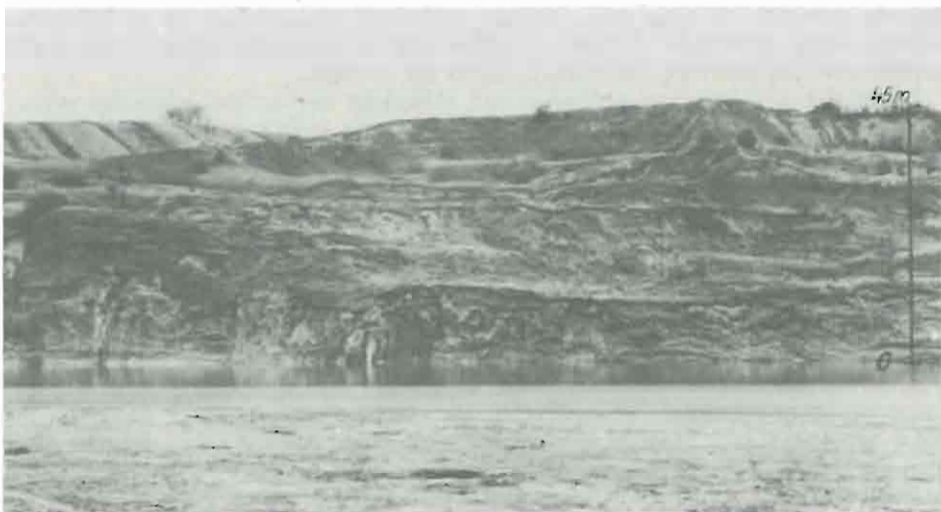
Portion of the great slide on the San near Krzeszów; watered contact surface between the Krakowic clays and the Quaternary deposits is one of the reasons of high activity of the slide
