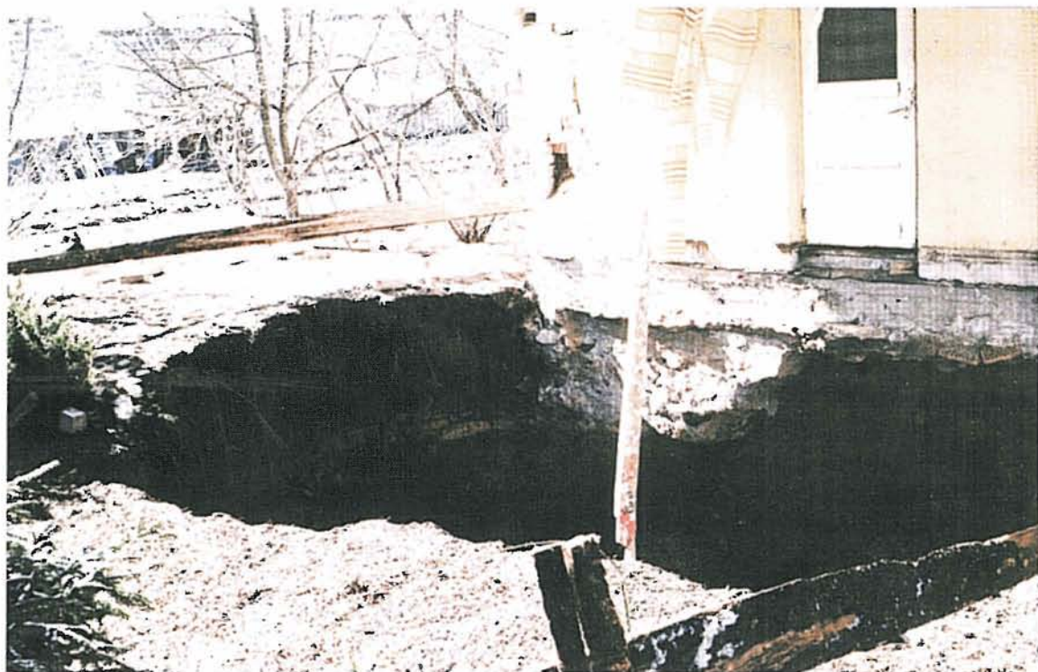
Fig. 5. Part of a house, after falling into a sinkhole 3–4 m wide and 5 m deep in Naciūnai village in April 11, 1997
