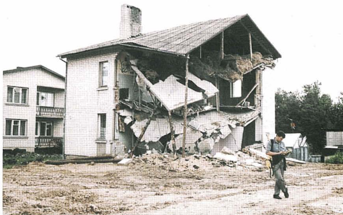
Fig. 3. Sinkhole appearance, with consequent damage to two buildings on June 15, 1999
