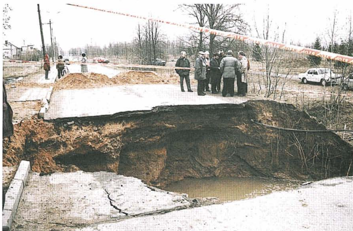
Fig. 2. The new sinkhole which suddenly opened on the Panevėžio Street, Pasvalys on March 5, 1997
