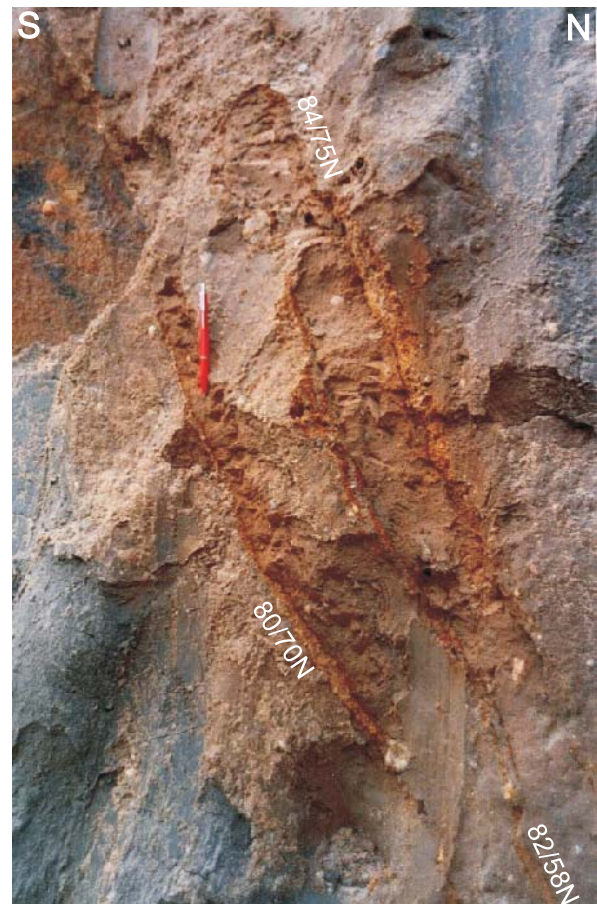
Fig. 14. Glaciotectonic thrust in till of the basal layer in NE part of pit (central part in Figure 9)
