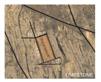
Fig. 8. Rectangular elementary block of intact rock in the limestone zone
