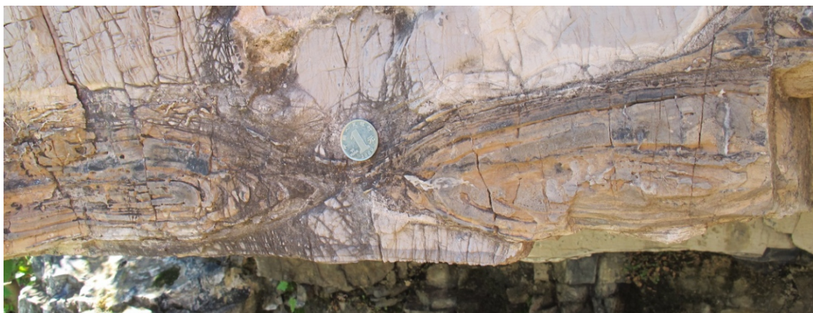
Fig. 3. Weathering of a diagenetically formed structure, resembling nodules
