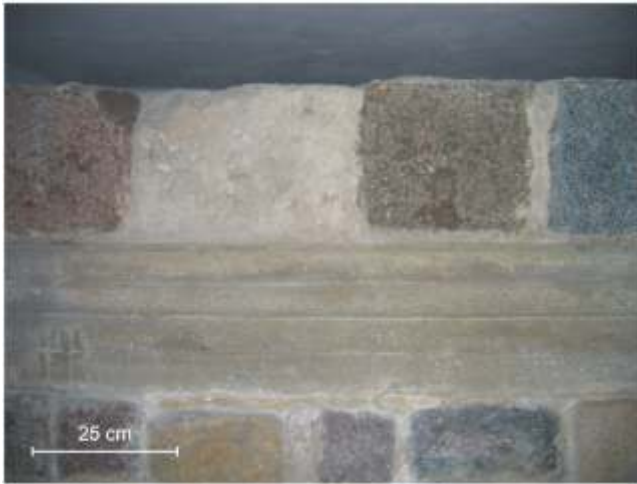
Fig. 6. Poznań, Ostrów Tumski; the basement of Poznań cathedral; a piece of pillar II of the Romanesque church; starting from the upper left corner: granite, calcareous sinter, granite, granite, in a large slab of sandstone from Brzeźno
