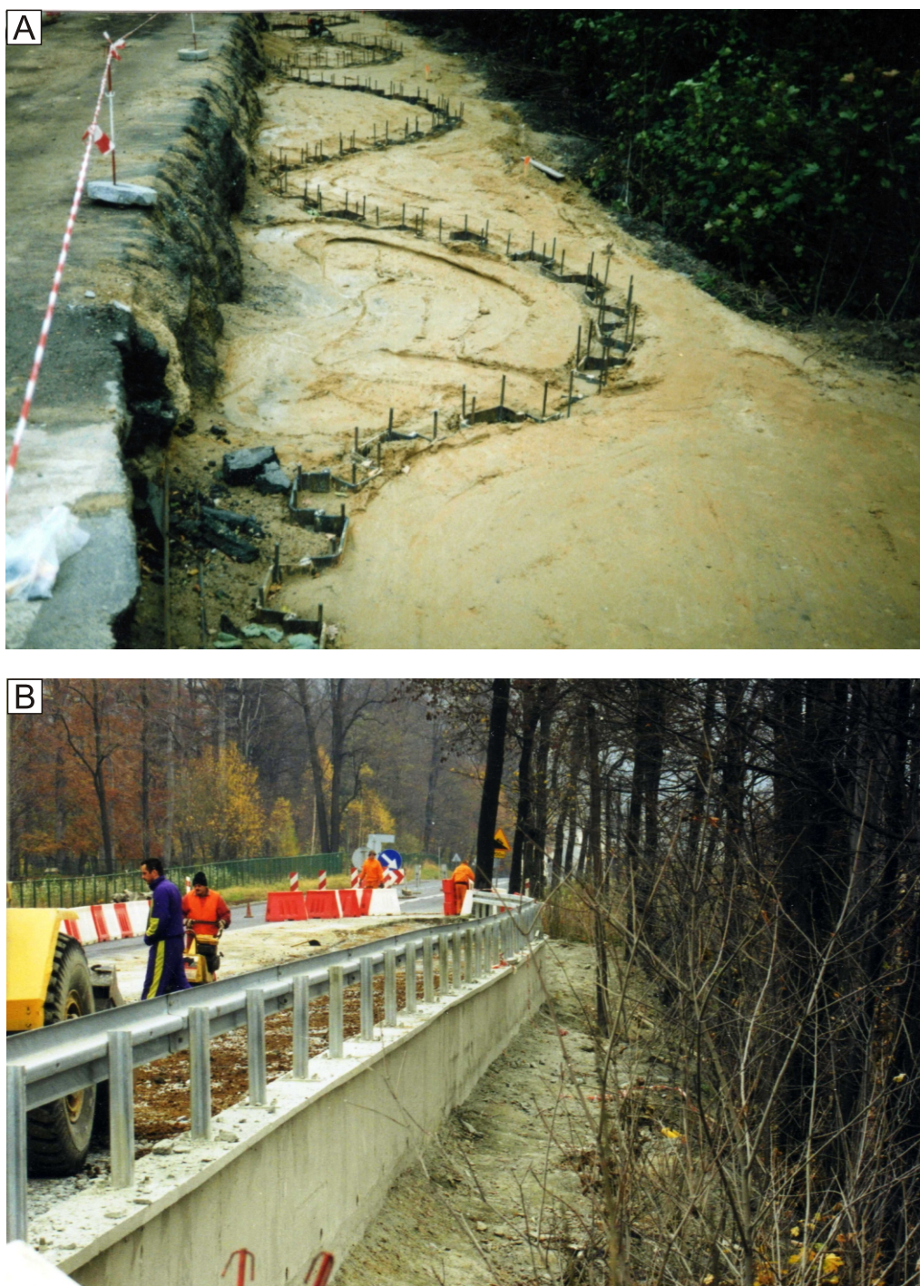
Fig. 13. Wavy buttress stabilising slope failure and widening the road from Figure 12
